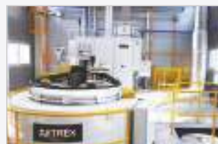
Gas Nitriding furnace
